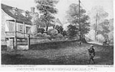
Somerindyke House on Bloomingdale Road near 75th Street
